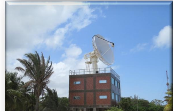
4: 7.3m Installed and Operational
