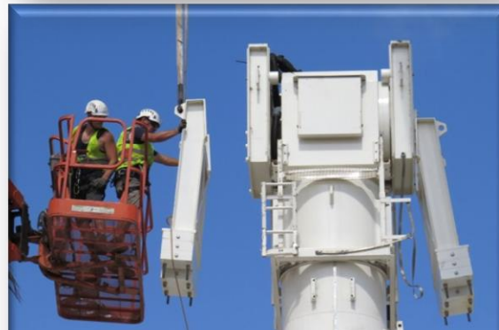
3: Counterweight Assembly on Pedestal
