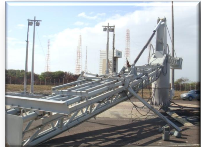
CLA Medium Size Rocket Launcher – LPM Damaged → 2015 Brazil Northeast – Alcântara / Maranhão State
