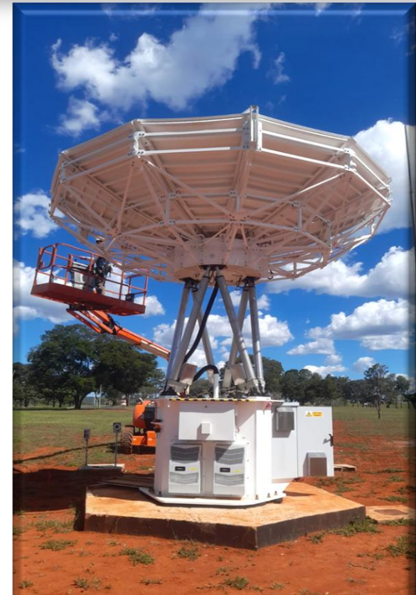
3: Lessônia Antenna Installed
