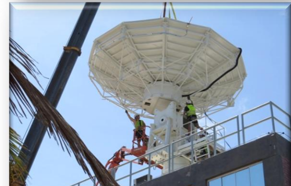
4: Reflector Assembly on Pedestal
