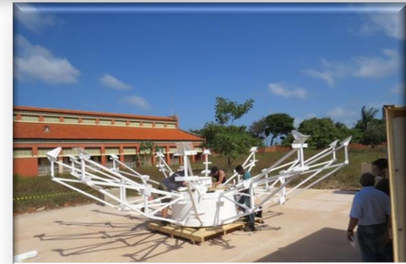
2: Reflector Structure Assembly Support
