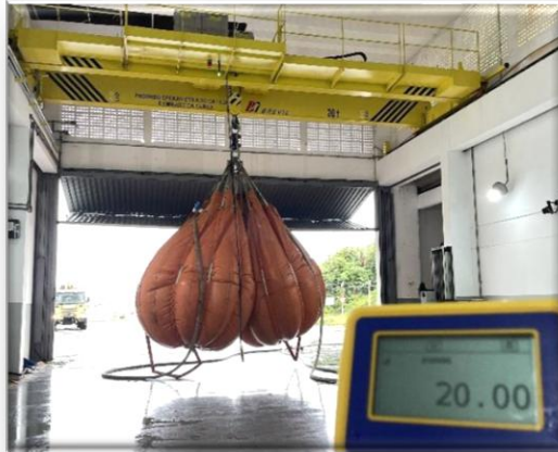
Testing of the 20-Ton Overhead Crane using water as load.
