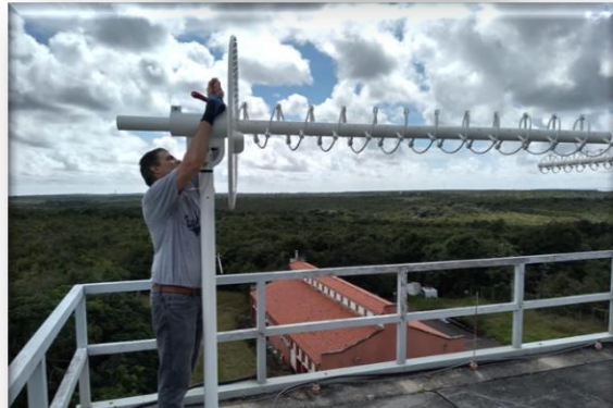
3: Antenna Installation
