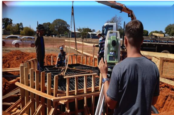
2: Antenna Block Concrete Structure
